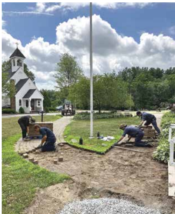
Despite the summer heat, the Brothers removed the old walkway and installed a beautiful new one.
