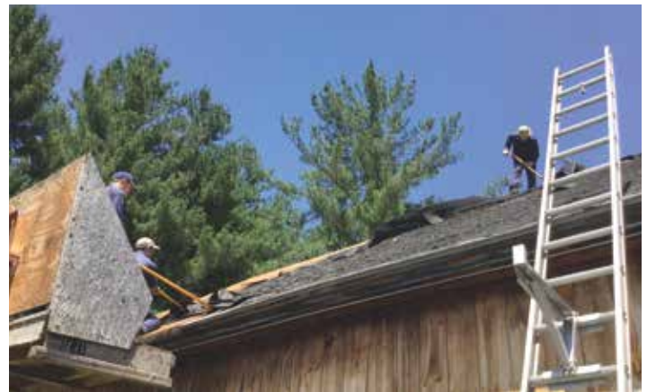
Brothers remove shingles and replace the plywood before re-shingling the pole barn seen at left.
